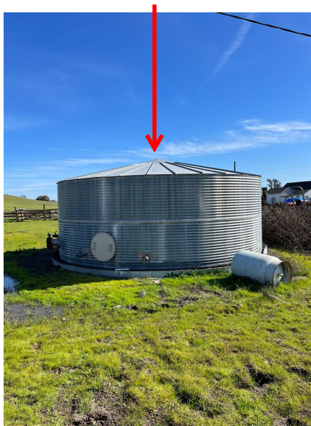
*NOT INSPECTED OR TESTED* Corrugated Steel Storage Tank
